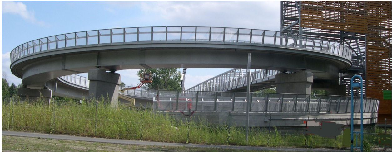
Spiral ramp in Longueuil
