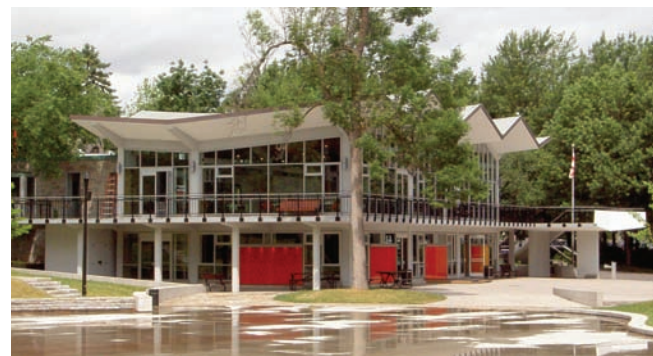
Renovated Beaver Lake pavilion
