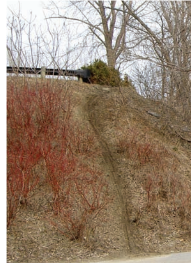
Damage caused by mountain bikes
