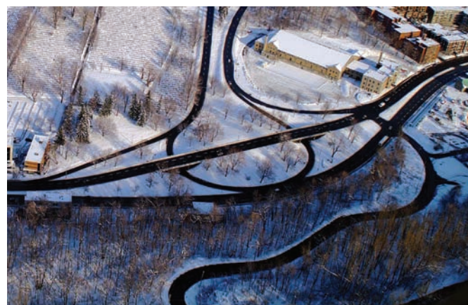
The reconfiguration of the Côte-des-Neiges-Remembrance interchange will simplify access to Mount Royal Park.
