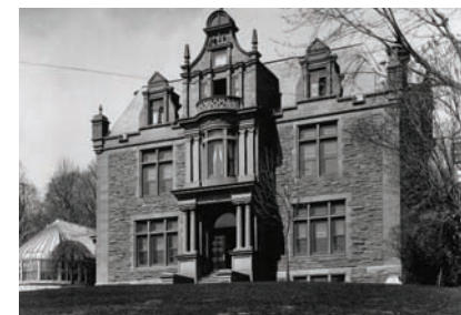
W.W. Ogilvie's residence, "Rosemount," Rue McGregor, 1894 (since demolished)
