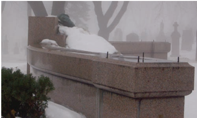
Commemorative monuments are suffering damage and some of their significant components are being lost.
