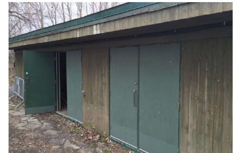
Station d'épuration, Jonathan Cha, 2016.
