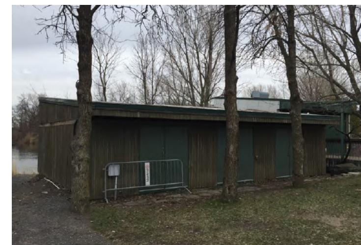
Station d'épuration, Jonathan Cha, 2016.
