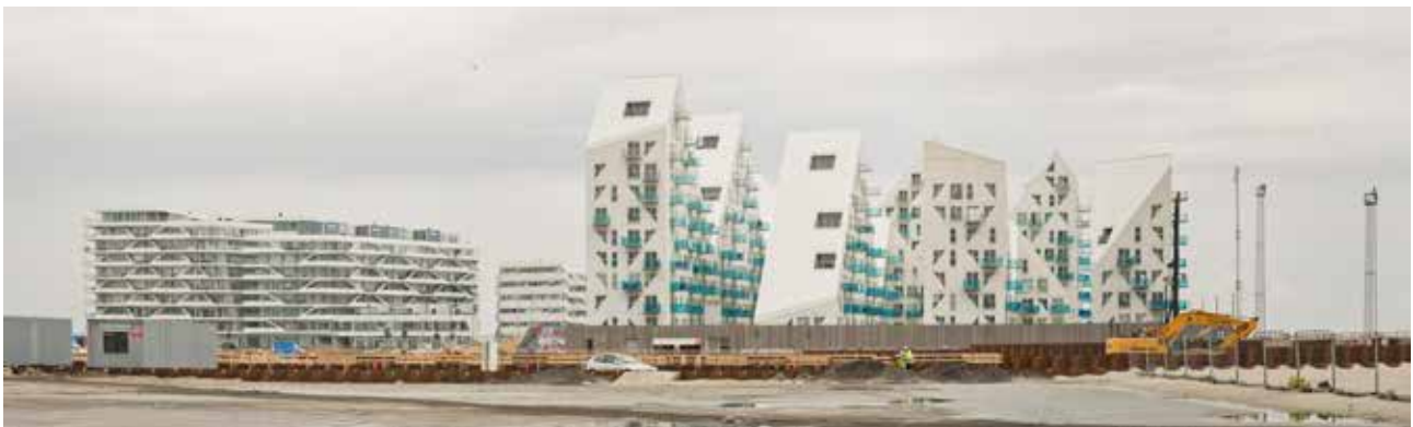
Photo 4.3 Brownfield recycling with ongoing construction
