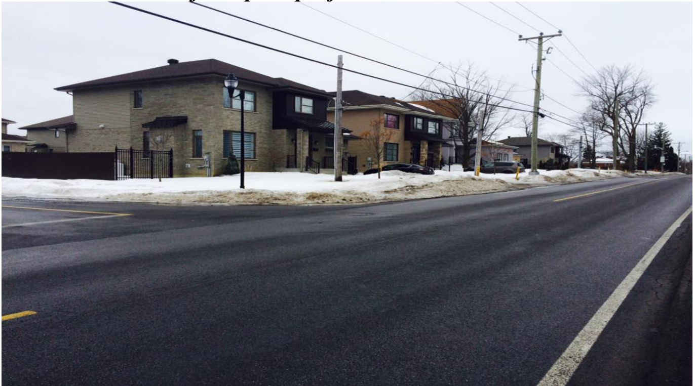
Gouin Boulevard after “pilot project”
