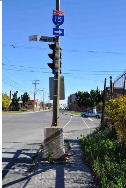
Issue 4: Traffic light centered on sidewalk impedes pedestrian flow
