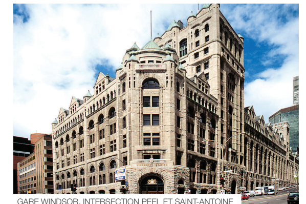
GARE WINDSOR, INTERSECTION PEEL ET SAINT-ANTOINE
