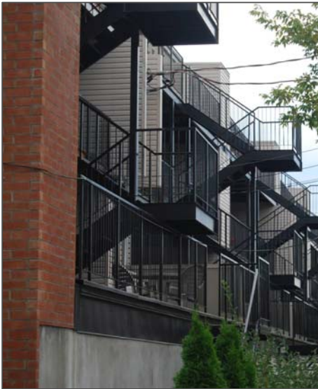
Residential building Parc-Extension Neighbourhood
