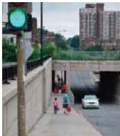
Figure 18b. The Girouard Viaduct Source: CEUM 2011.
