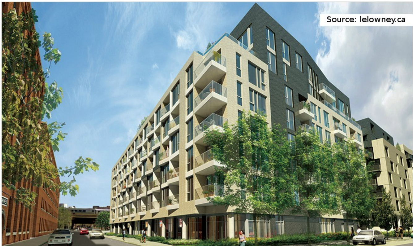
Figure 3. Final Version of Lowney Phase 8 with Phase 9 in Background
