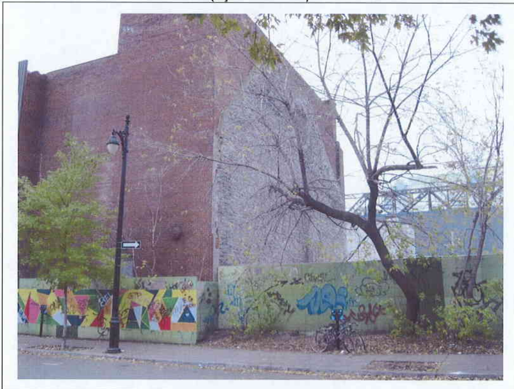
Photo No. 2 – Façade nord.
