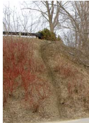
Damage caused by mountain bikes
