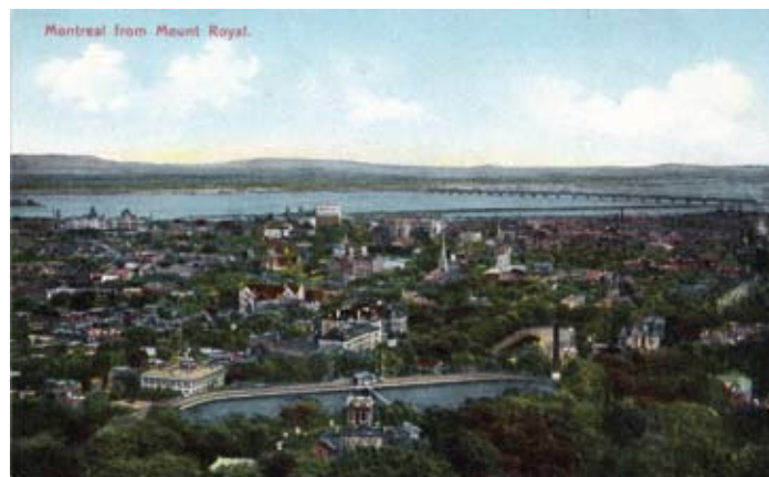
Postcard showing the McTavish reservoir before it was covered with a concrete slab in 1947.
