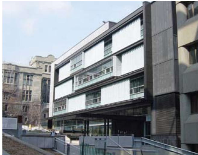
Trotter pavilion at McGill University
