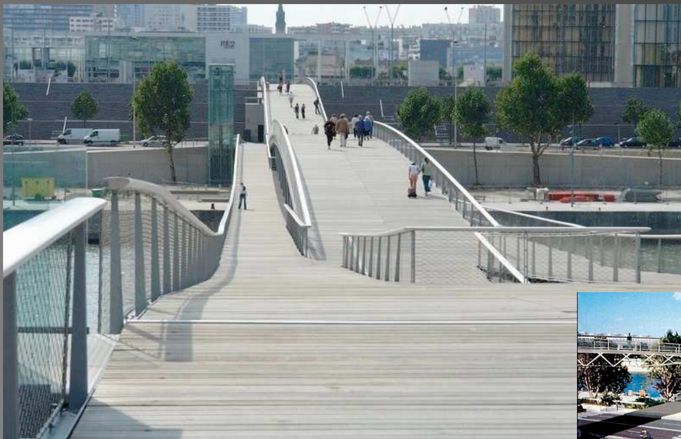
Passerelle Simone de Beauvoir, Paris
