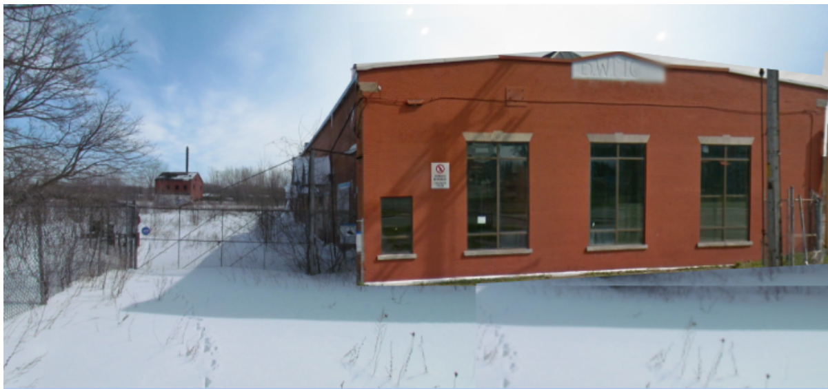
Fig. 3 - Dominion Wire Manufacturing Ltd
