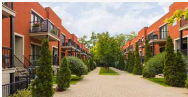
View of the entrance to a multi-unit courtyard grouping, accessible from rue Bossuet
