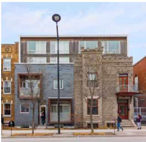
Addition of a floor onto an existing building.
