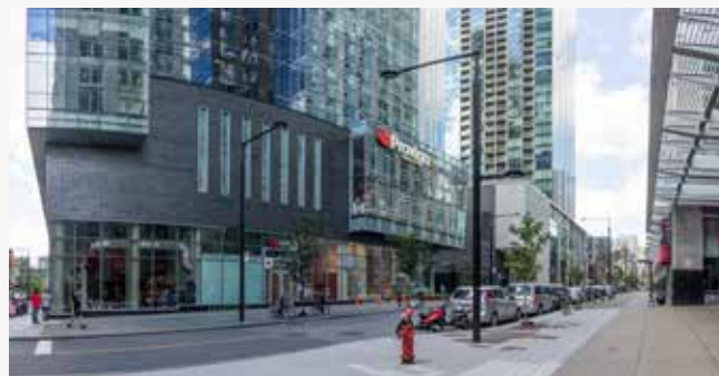
Tower podium containing commercial space, seen from rue Drummond.
