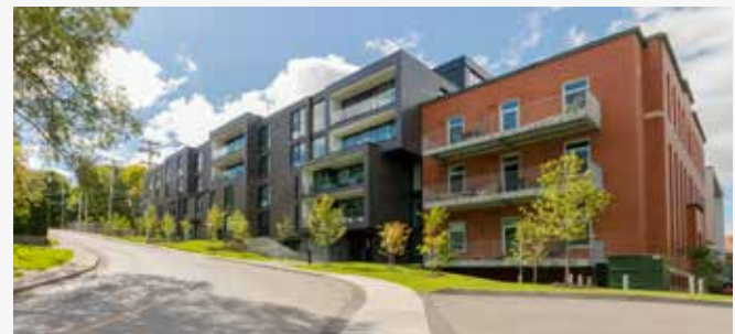
Original building and new volumes, from côte du Vésinet.
