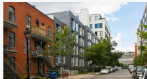
Construction of a new volume provides gradation between the industrial buildings and typical Montréal plexes.
