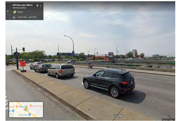
Figure 52 | The current intersection of Decarie and Jean-Talon (Google Street View)
