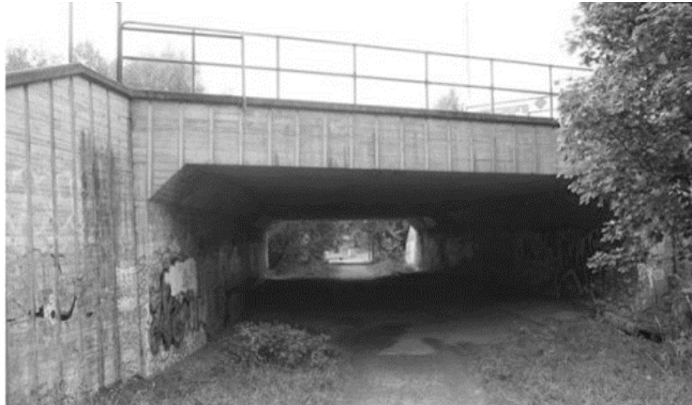
Figure 45 | Ammarud Viaduct in the Netherlands before renovation.
