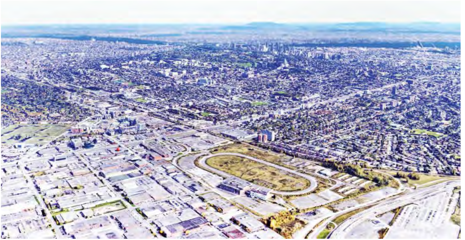
Figure 24 Aerial view of Hippodrome with Décarie and TMR in the background (BANQ)
