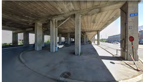
Figure 38 | A40 Underpass (Google Street View)
