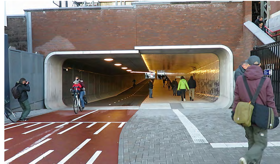
Figure 46 | Ammarud Viaduct active underpass after renovation. (Reprogramming the City)
