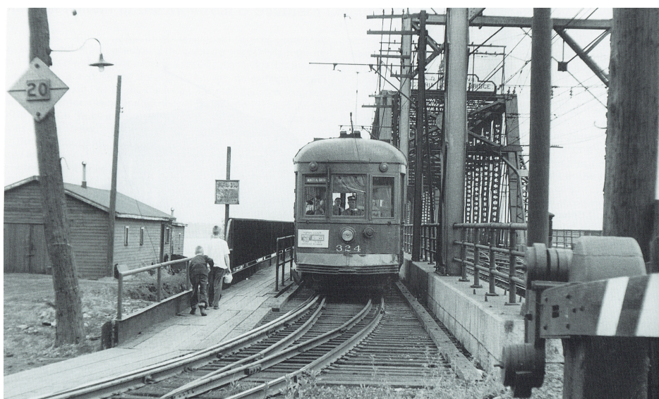
Tramway traversant le pont Victoria, 1955 (J.R. Thomas Grumley, Montreal & Southern Counties Railway Co. , p. 24)
