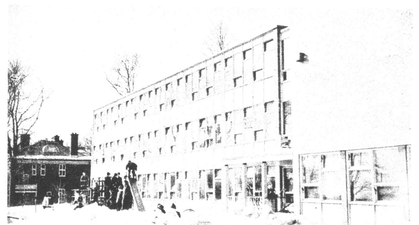
School was started in a house in 1930. Parents gave $100,000 for deposit on new building opened in 1957.
